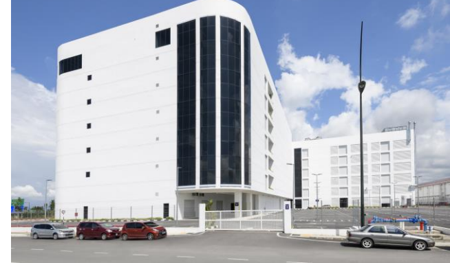
Penang, new production site
