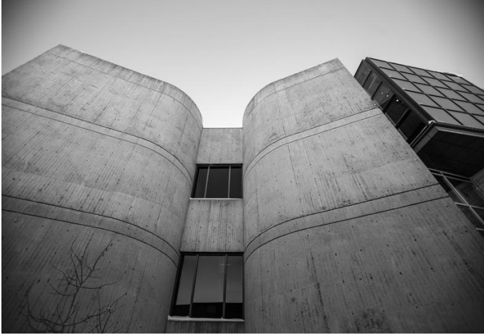
The brutalist architecture of Contemporary Calgary. Courtesy Gerard Yunker and Contemporary Calgary
