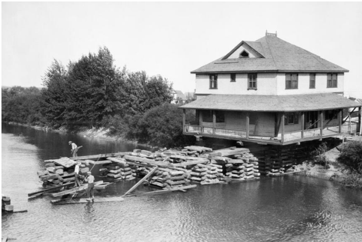
Superintendent Burton Deane's house being moved to the east side of the Elbow River, 1929. By W.J. Oliver. (CU193485) Courtesy Digital Collections, University of Calgary
