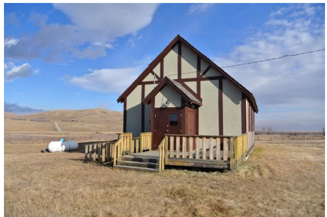
St. Aidans Anglican Church. Courtesy LocationHub
