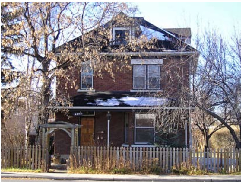
Patrick Ranch House - 37 Street W.
