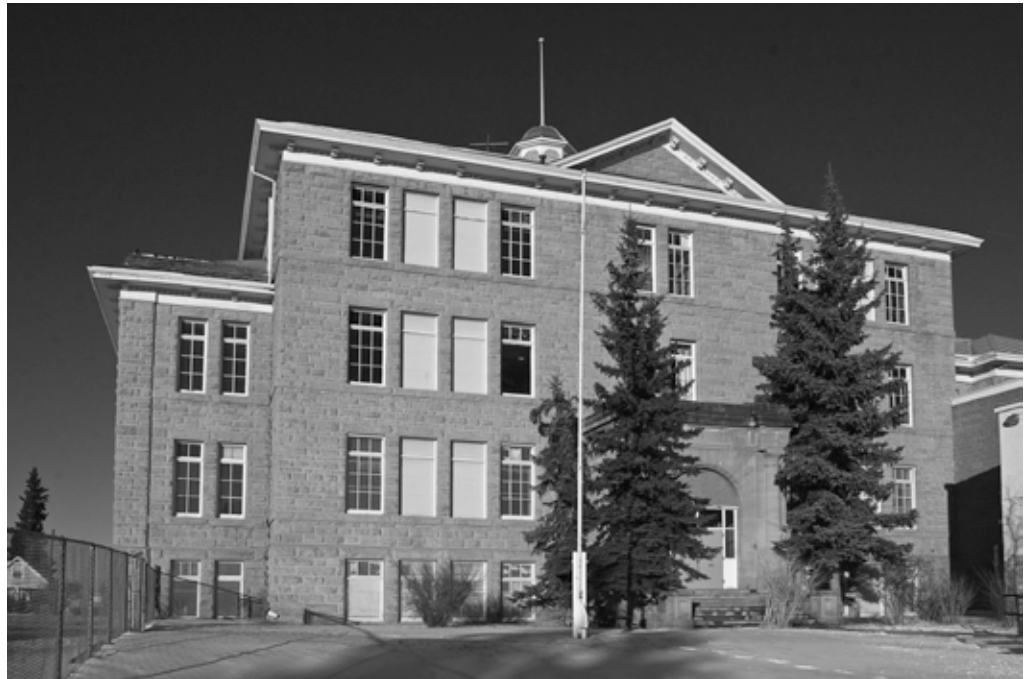
King Edward School, South Facade Today
