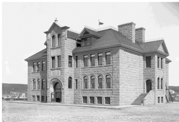
Riverside School was demolished in 1968 after a fire gutted the building.
