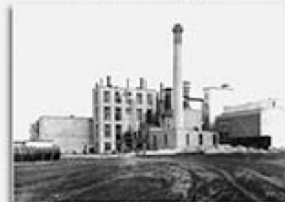
Calgary Brewing and Malting Co. building, ca. 1905-1906
