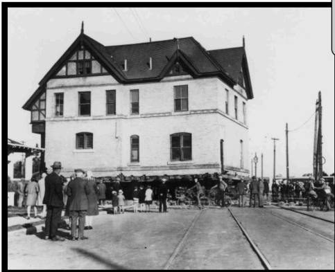
Costigan house built in 1895 at 1 Street and 17 Avenue SW, moved to 219 - 17 Avenue SW in August 1928 Col. Samuel B. Steele once lived in this house Courtesy Glenbow Archives NA-2186-10
