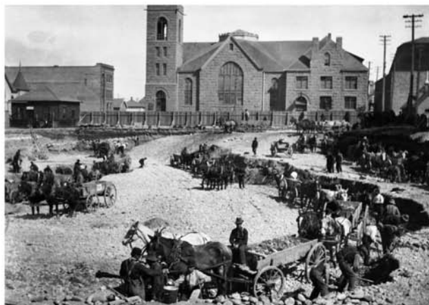
Excavation for Hudson's Bay Company Store (ca. 1911) 7th Avenue and 1st Street Glenbow Archives NA-2732-3
