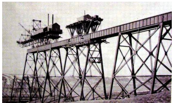
Construction on the Lethbridge Viaduct, ca. 1908. Courtesy John Unsworth
