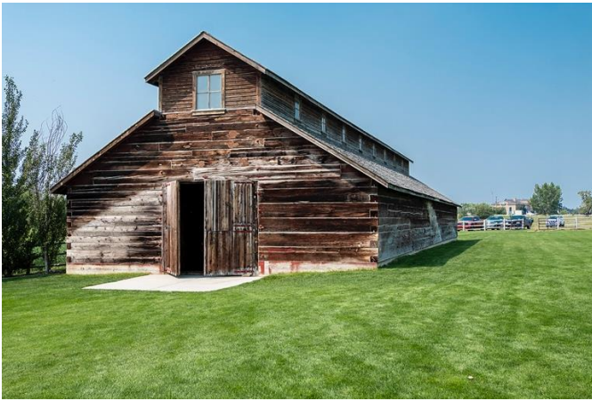
Building on Canadian Pacific Supply Farm No. 1. Courtesy Walt DeBoni
