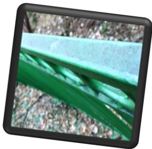
Top Rails Not Painted!
