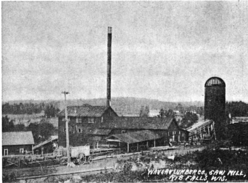
Wausau Lumber Company. Left to right, blacksmith shop, with the mill pond in rear, saw mill and conveyor going up to slab burner.
