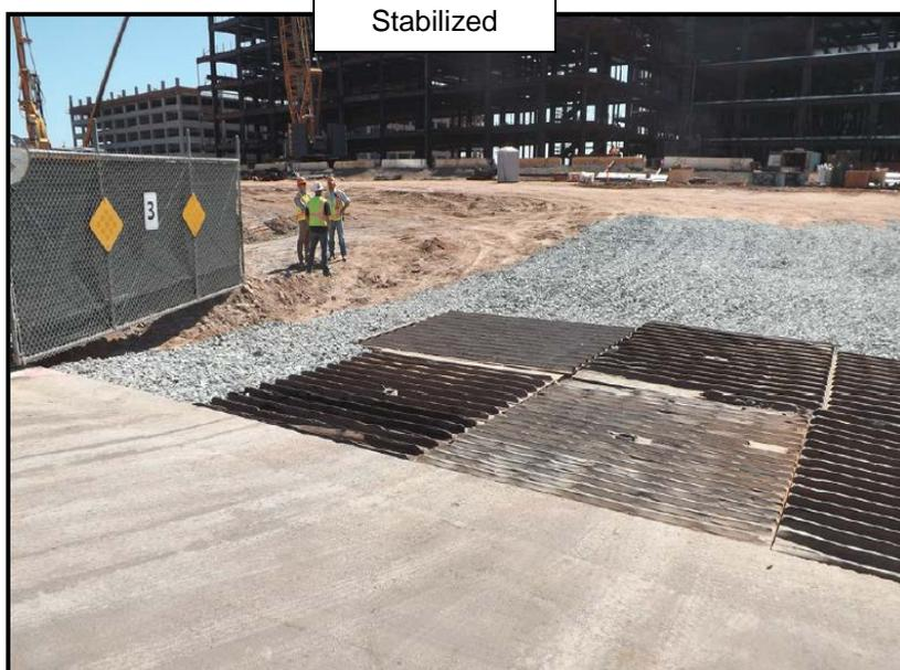
Because stabilized entrances/exits are only moderately effective, this particular BMP should be used in conjunction with street sweeping, and should undergo routine inspection and maintenance.
