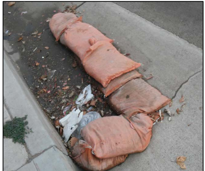
Chevrons require periodic cleaning and maintenance.
