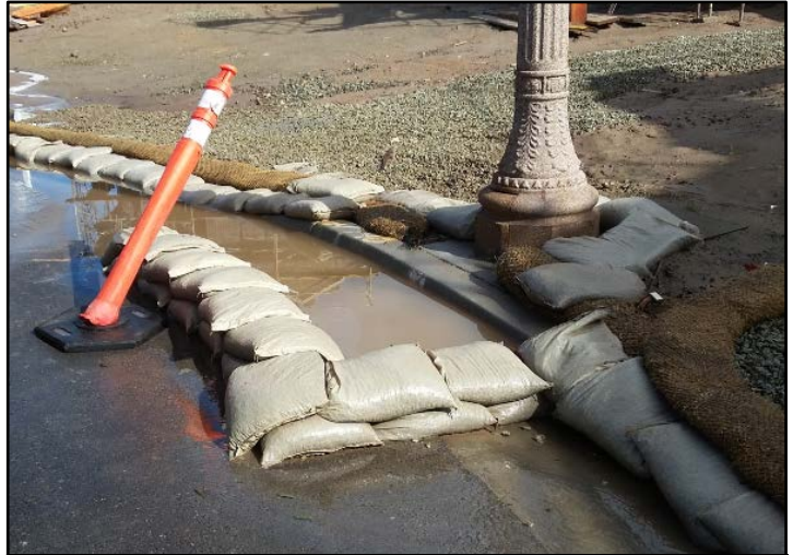
Chevrons help filter sediment from stormwater runoff.
