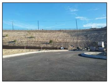
An example of wood mulch applied to a slope to prevent erosion.
