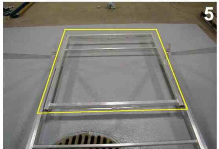
5. place the top frame at the un-bolted ends of the H-frame the welded strap should be on the bottom when it is set in place
