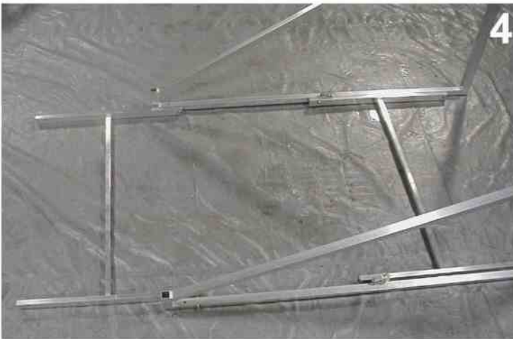
4. mount the 2nd H-frame to the water end of the lift. Use picture #3 for the bolting detail, the bolts are the same.
