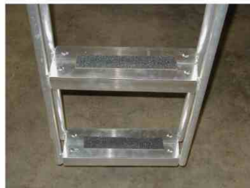
Apply self adhesive anti-slip tape
