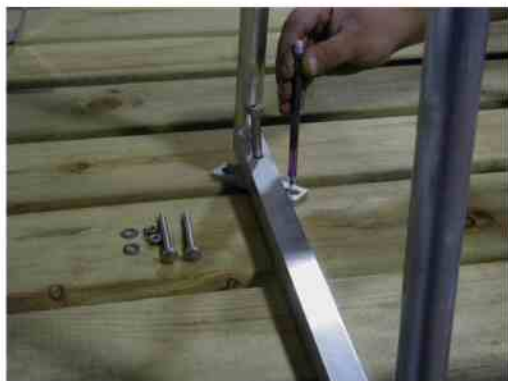
Place mounting plate under ladder. Drill 3/8" hole through deck for mounting bolt if necessary. Mark oblong holes and drill 5/16" holes
