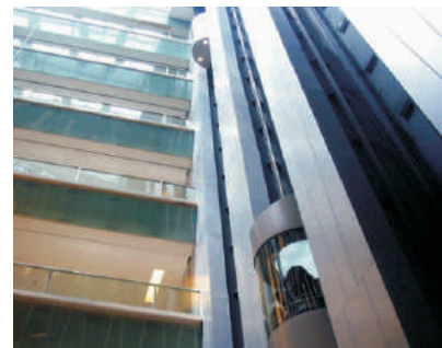
Elevator Industrial field
