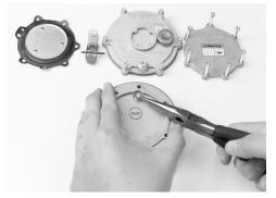
13. Holding the valve pin in place, turn the body cover plate over. Place the valve pin spring (16) over the valve pin with the larger diameter end of the spring resting against the plate. Compress the spring and secure it in place by installing the "E" ring (17) retaining clip to the valve.
