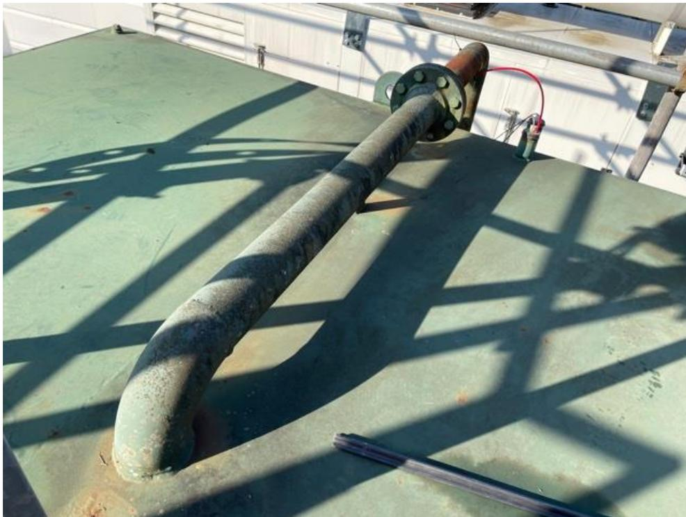
Fig 16. Fill Pipework
