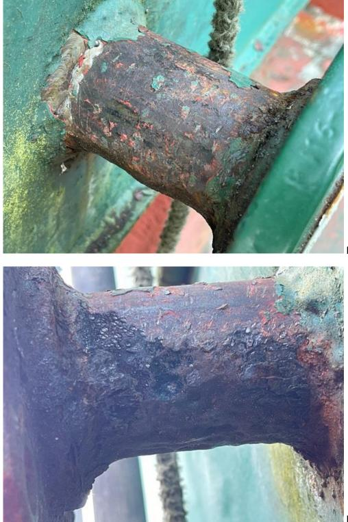
Fig 9. Outlet Nozzle Close-Up
