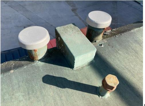
Fig 17. Tank Vents & Dip
