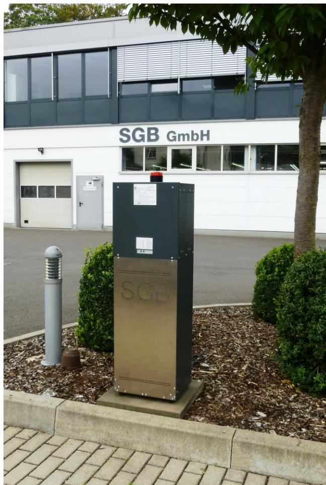
**Leak detection unit LDU14:** 100 % continuous monitoring of up to 12 tanks and 12 pipes by pressure leak detection technology. Tanks as well as pipes are monitored separately by two pressure leak detection systems based on air. In case of pressure loss an alarm starts immediately before any product can pollute the environment. LDU14 is in accordance with class I of European standard EN 13160.
