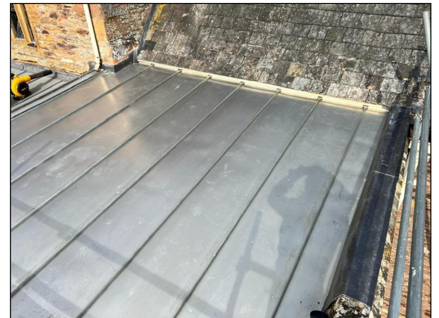
New stainless steel roof coverings and flashings installed in line with other areas of the church roofs.
