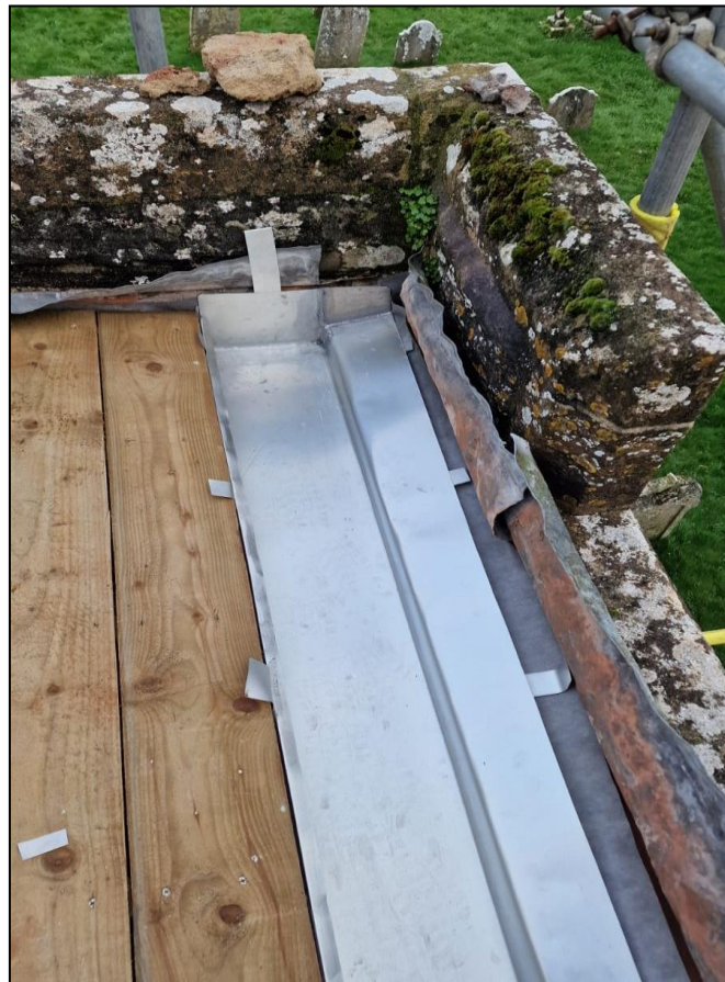
Replacement timbers and aluminium rainwater systems installed.
