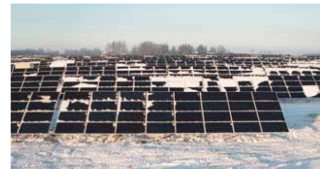
Figure 1 - Soiling mismatch
