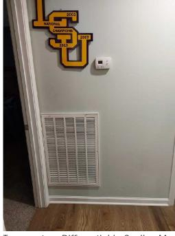
Temperature Differential in Cooling Mode 20° F -- Temperature difference between return air and the register should be between 14F and 22F. This unit is operating at the high end of the standard.
