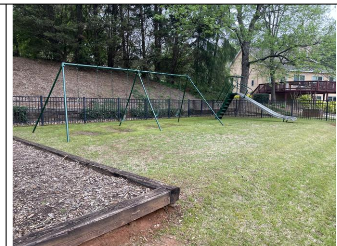
Wall around play area and outside fence
