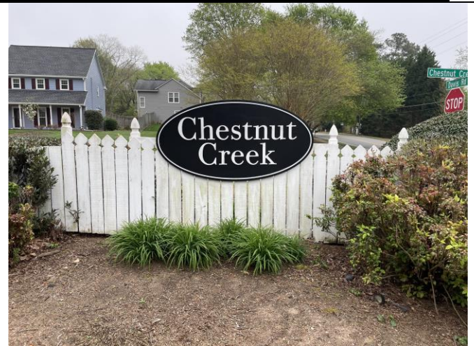
Entry monuments require routine painting
