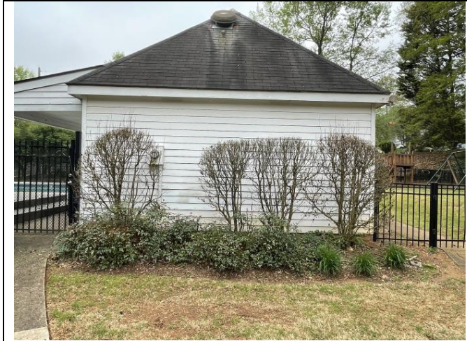
Example of the siding
