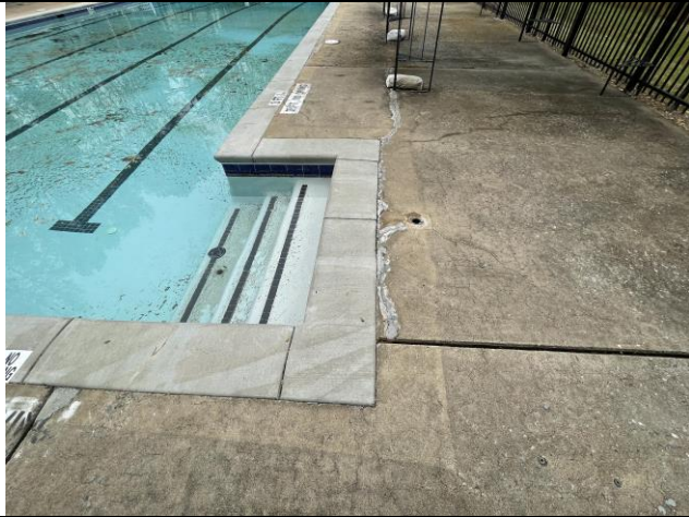
View of the pool with new edge and pool surface
