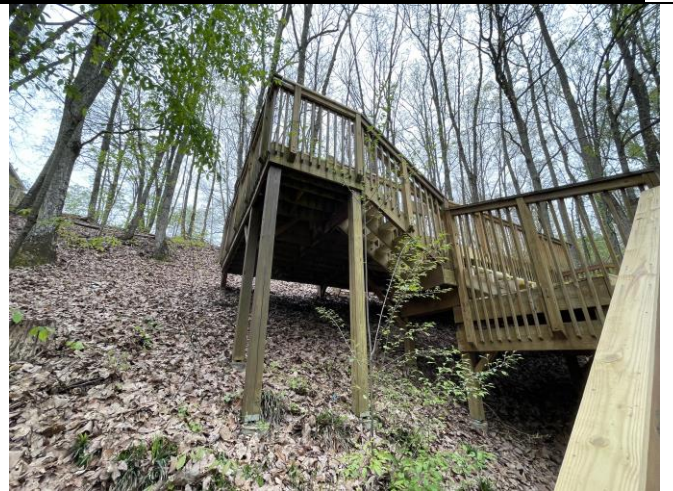
View of tennis observation deck structure
