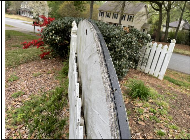
Weathering on the sign mounting board
