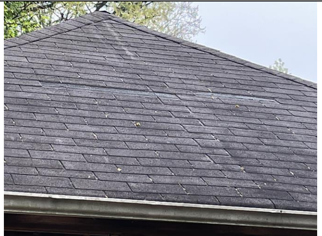
Pavilion roof with mission shingles
