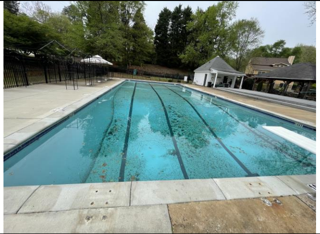
Another pool shot with replaced decking at left
