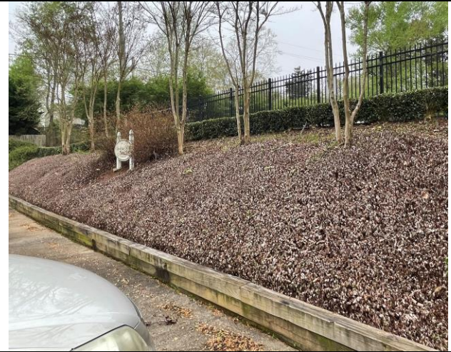
Wall at parking area
