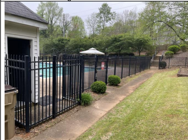
Six-foot metal fence around the pool
