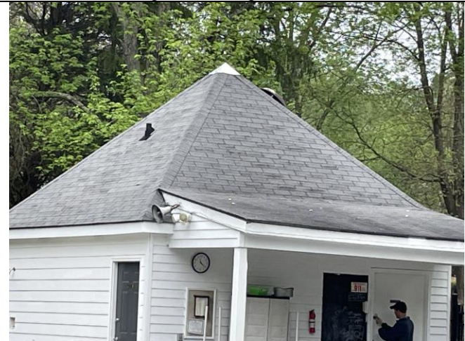
Another view of poolhouse roof
