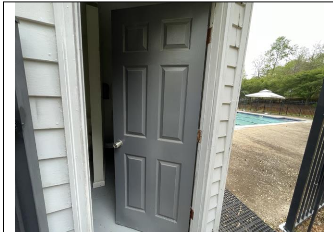
Ladies bathroom door is interior rated hollow core
