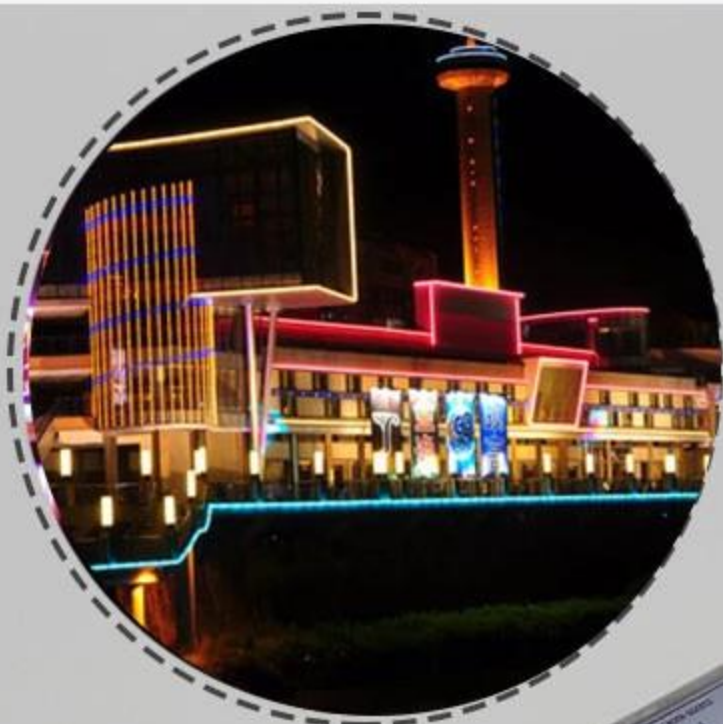
Building outline lighting
