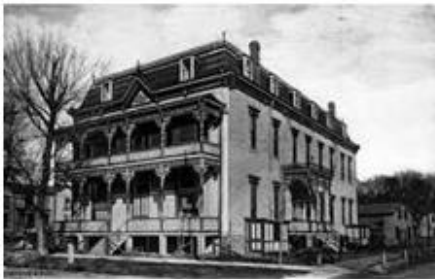
Original MPI Building
