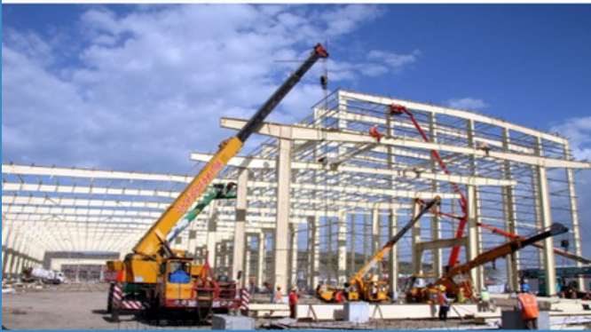
Structural fabrication and erection
