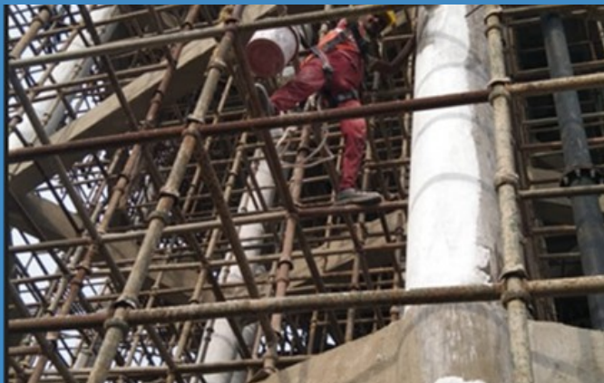
City supply - WTP inlet maintenance
