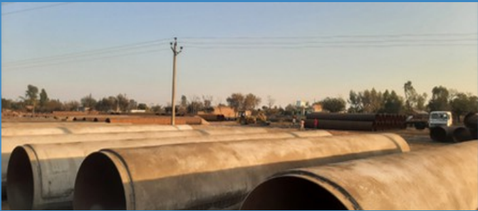
Guniting / Concrete Coating on irrigation pipeline – JayPee Associates – Rewa MP
