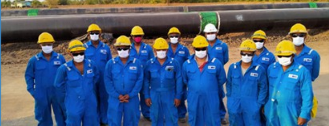
Gas Pipeline Wrapping & Coating – at IBCI -Thailand
