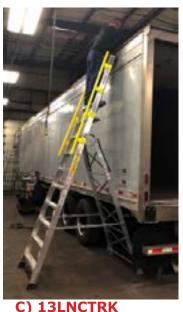
Free standing ladder allows stable working access to the higher truck exterior.
