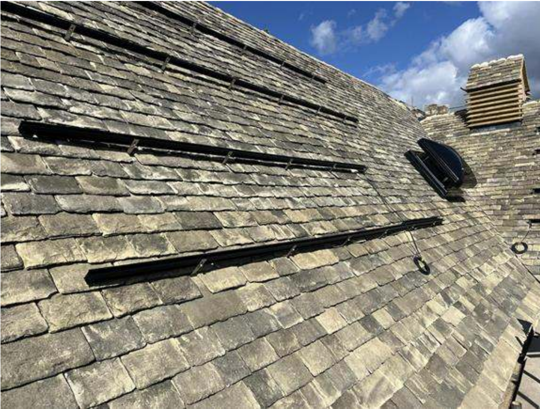
Courtyard – South Facing
