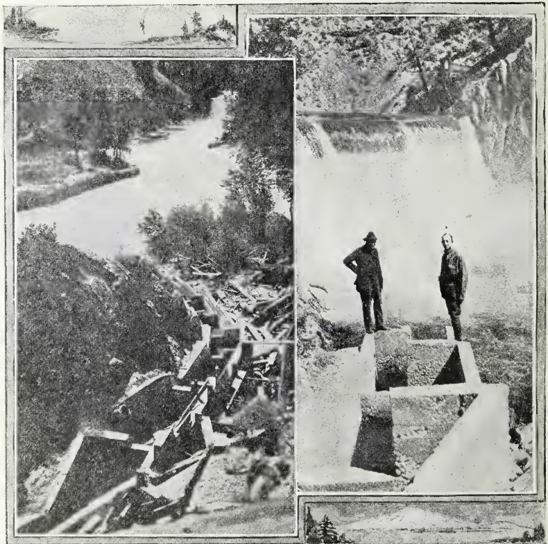
Sectional Views of the Concrete Fishway Constructed Over the Sunbeam Dam During the Spring of 1920
