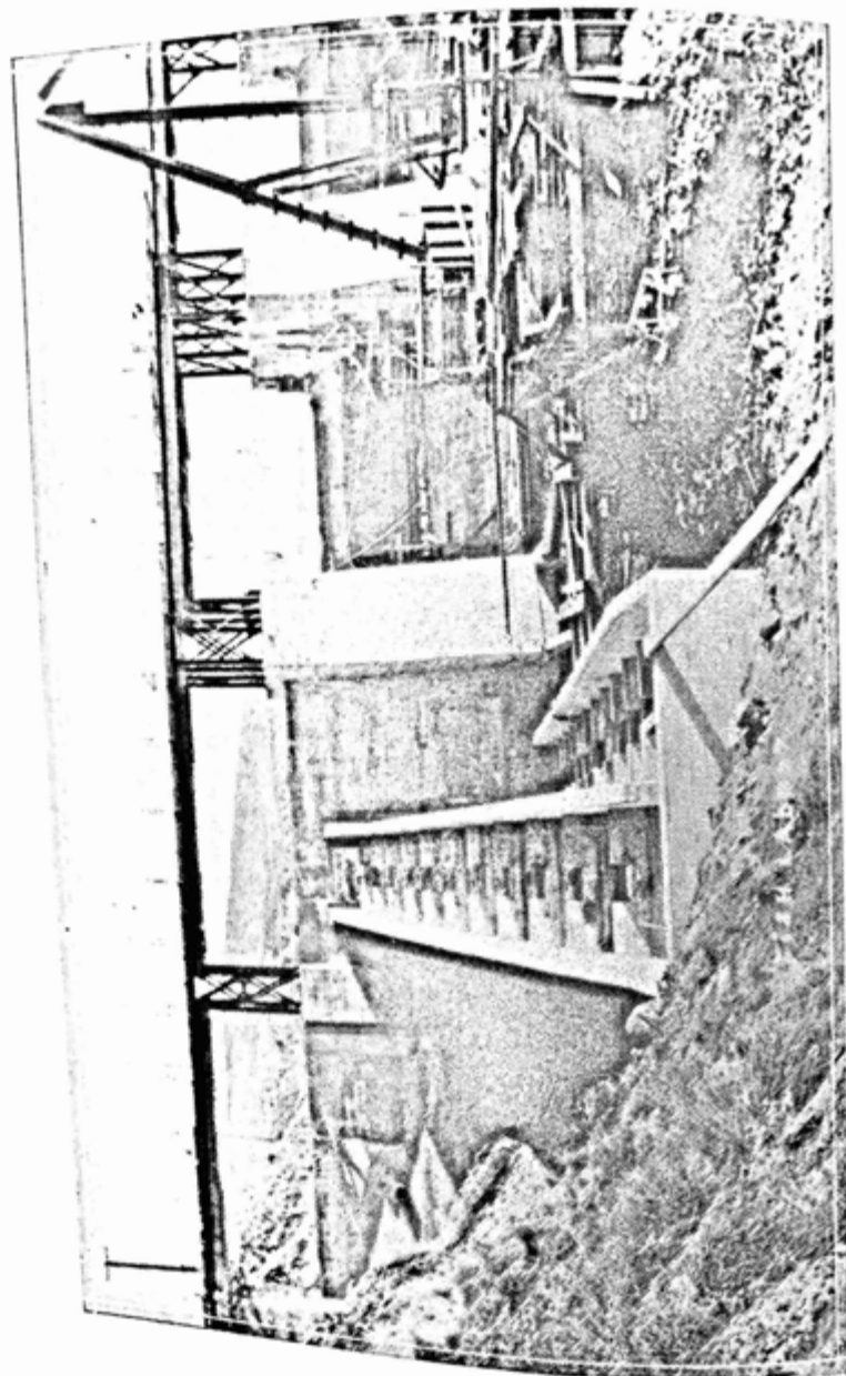
FISH LADDER IN THE CLEARWATER DAM. THIS TYPE BEING ONE OF THE MOST PRACTICAL EVER CONSTRUCTED IN IDAHO
