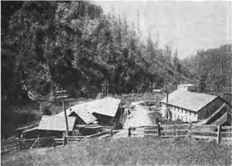
Kalama hatchery. Covered rearing ponds on the left and hatchery on the right of the road.
