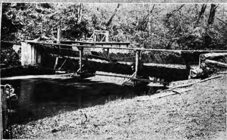
UPPER RACK AND TRAP AT THE GREEN RIVER HATCHERY
