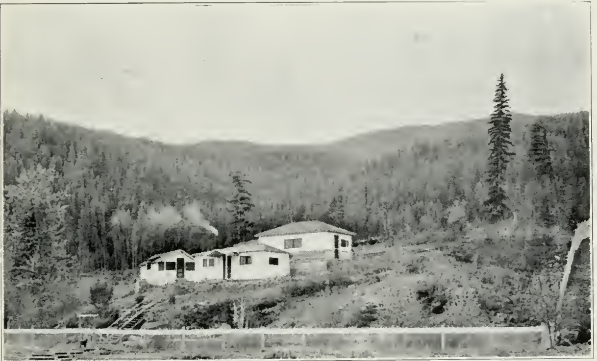
The photograph above shows the main buildings and a portion of the land under fence at the Swan Lake fur farm. The lower fence fronts on the lake shore. The experimental pens are located back of the buildings and the fence is so arranged that the fur-bearing animals may be controlled and conserved.
