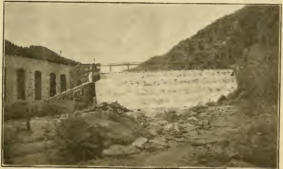
Here's a picture of the dam and a corner of the building of the Butte Anglers' Club fish hatchery at Divide, Mont., on the Big Hole River. The use of the building has been granted to the enterprising Butte club for use as a hatchery. The plant at Columbia Gardens, where game fish have been hatched from eggs supplied by the State Commission, and then distributed by club members and employes, will be discarded when the Divide hatchery goes into operation this spring.
