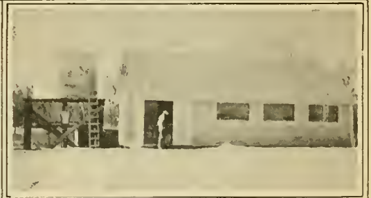
TANK HOUSE —LAKE GARBERSON—
