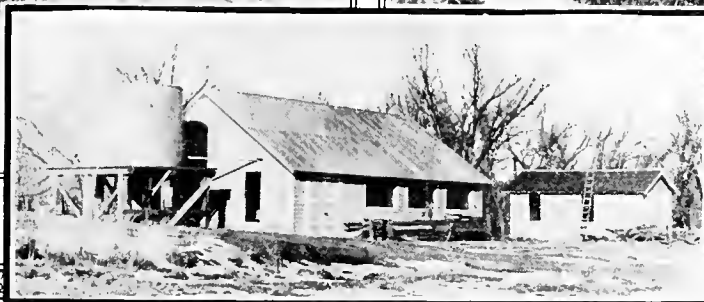
TANKHOUSE AND GARAGE
