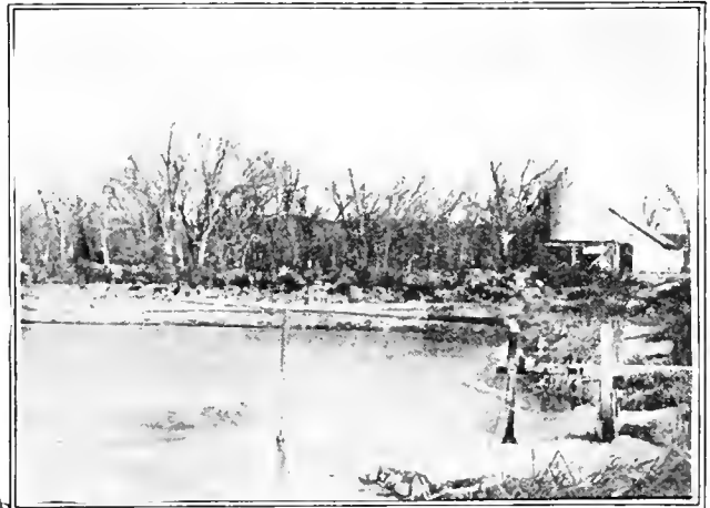
LOOKING TOWARD DAM SHOWING ARTESIAN WELL AND PORTION OF BUILDING
