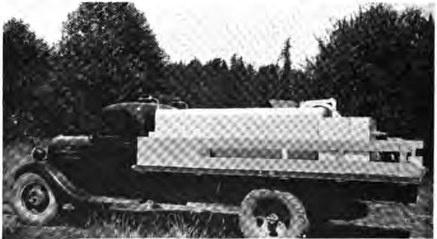
Mobile game fish tank carrier, 400 gallon capacity. In normal weather it is hoped that this new unit of the game fish planting division will be able to carry 150,000 small fry or 6,000 4-inch fish. Aeration is by water circulation.
