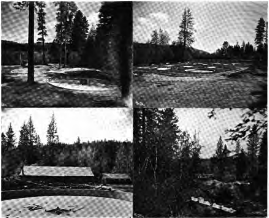
(1) Battery of standard concrete rearing ponds. (2) U. S. Bureau of Fisheries ponds. (3) Hatchery and garage, (foreground) section of standard 40-foot rearing ponds. (4) Water intake at new Spokane Hatchery.
