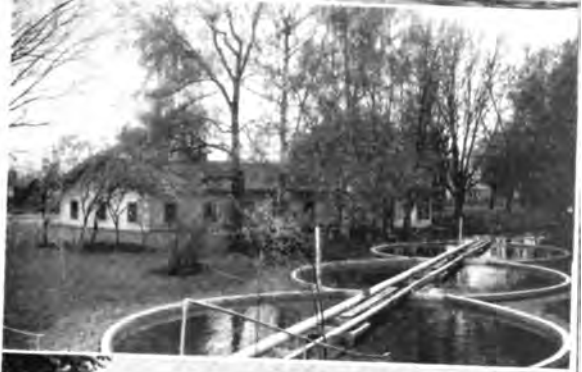
Walla Walla hatchery building and ponds.
