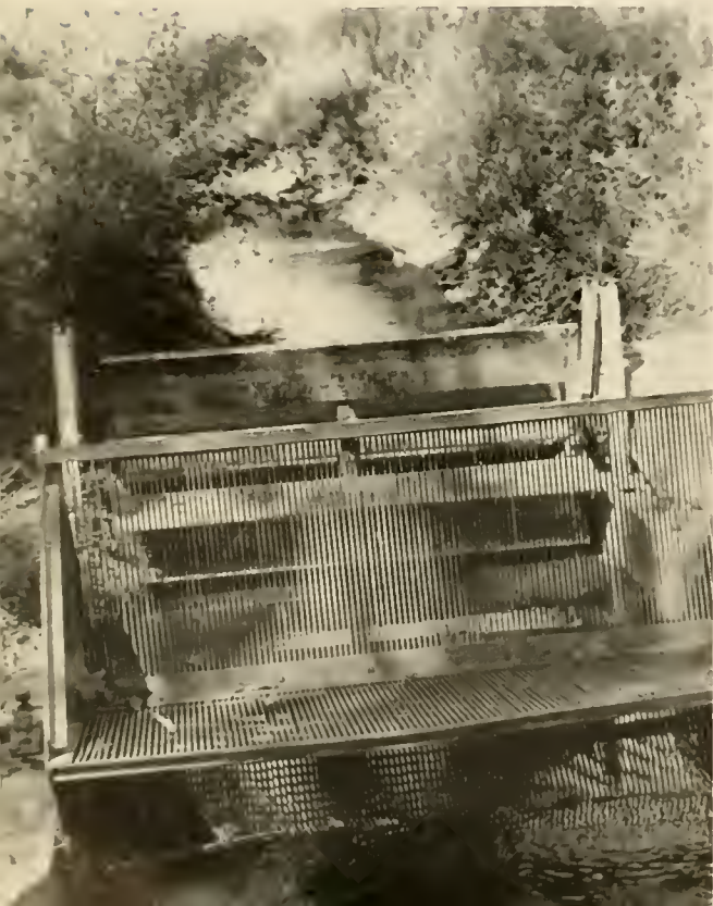
Oregon type fish screen with rotating grills—self-cleaning.
