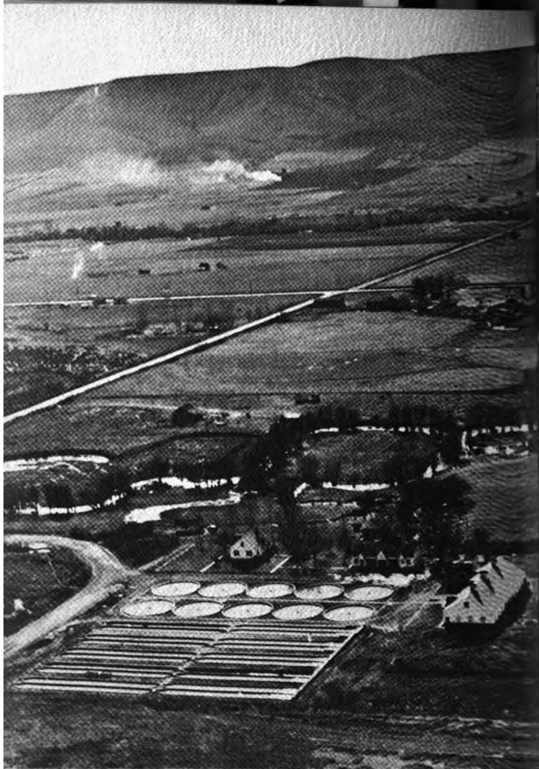
The trout hatchery at Yakima, Washington, one of the projects improved by the Construction Department during the biennium.
