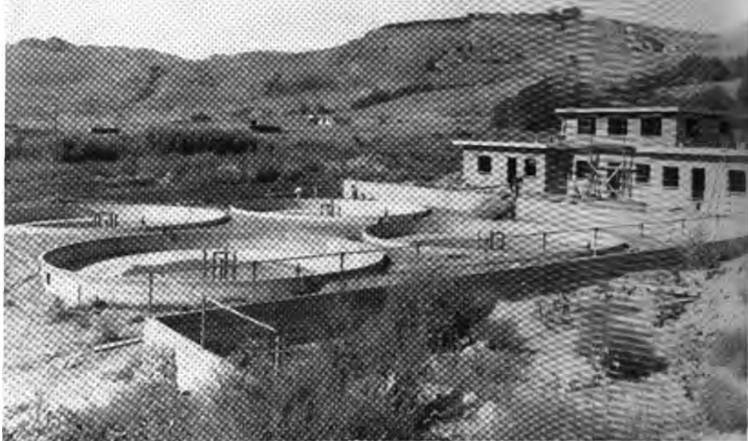
During the past 20 years, the Department's Engineering division has constructed modern trout hatcheries such as this one at Omak.
