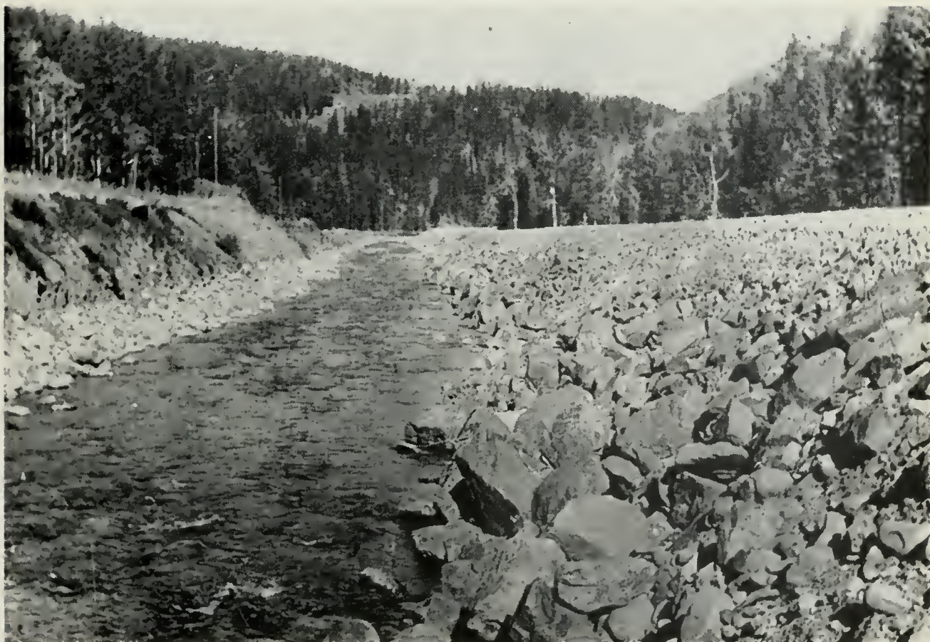
POOR STREAM HABITAT . . . Straightened to accommodate the highway at right.
