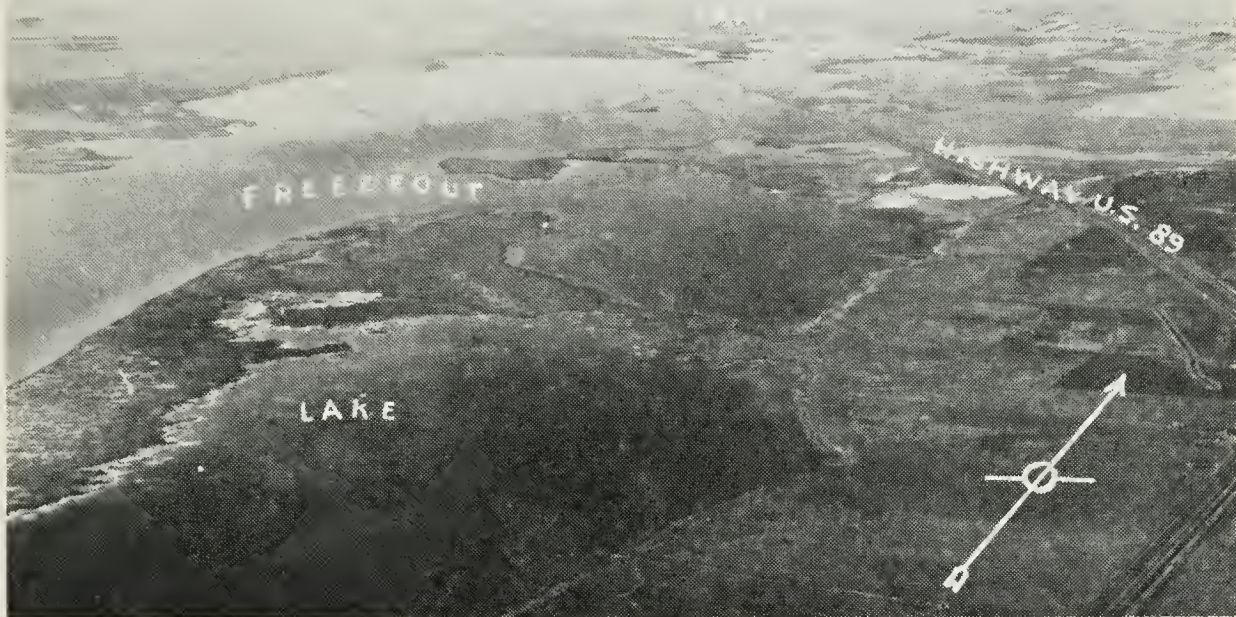
Construction of an outlet canal, representing the initial phase of development of Freezout Lake, was begun during the biennium.
