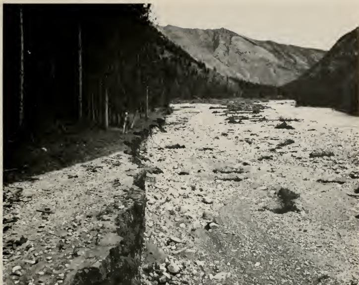
This is a portion of the North Fork of the Teton River following the June, 1964 flood. (Photo by U. S. Forest Service)
