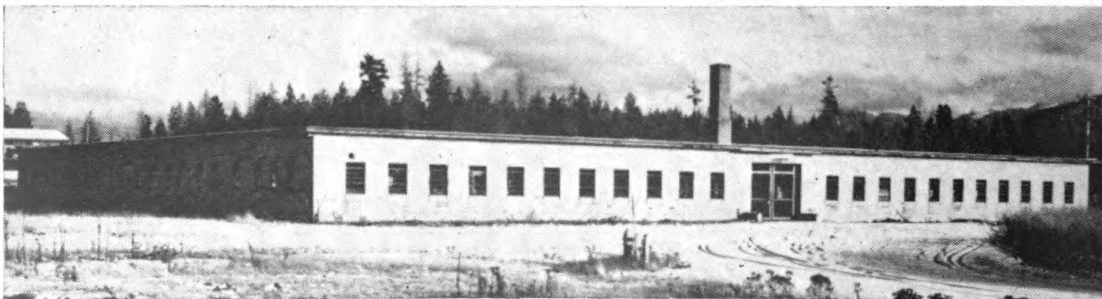
The brig, which formerly held unruly gobs, may be used for district warehouse by the fish and game department. Huge cement-floored building is ideal for storage and equipment dispersal center. Future plans call for conversion of Farragut Base into public recreation area.
