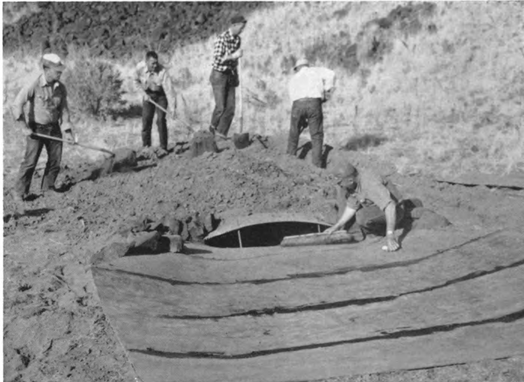
Fourteen self-filling, plastic water cisterns were installed during the biennium. These collect rain and snow run-off water making it available for birds during late summer and early fall.
