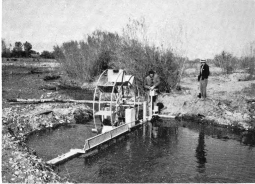
Fish screen on a Lemhi River irrigation canal.
