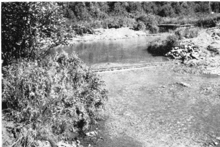
Granite Creek, tributary to Lake Pend Oreille, showing improvement work which enhanced the stream for kokanee and trout spawning. Two K-dams are shown.
