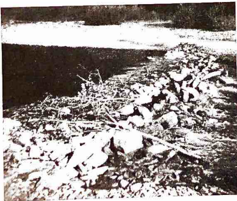
Small rock structures aid to provide pool space for trout. Beaver have utilized this effort for a dam of their own.
